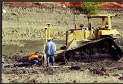
GPS guided dozers provided final grade accuracy
