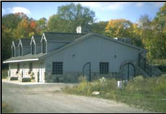
Completed Acacia Park CSO Basin
