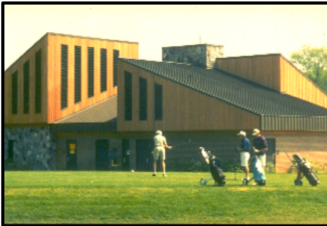
Completed Bloomfield Village CSO Facility
