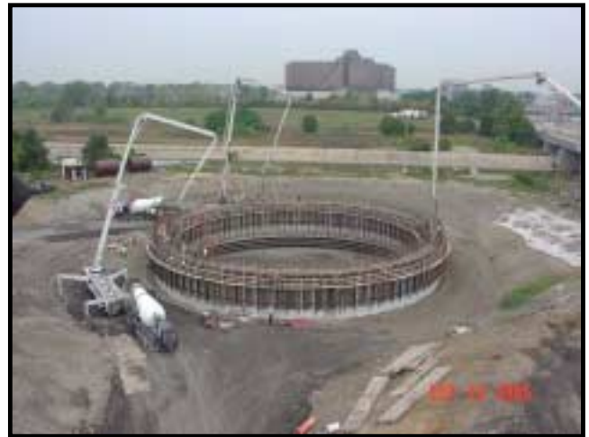
Construction of Capture Shaft at Greenfield Village
