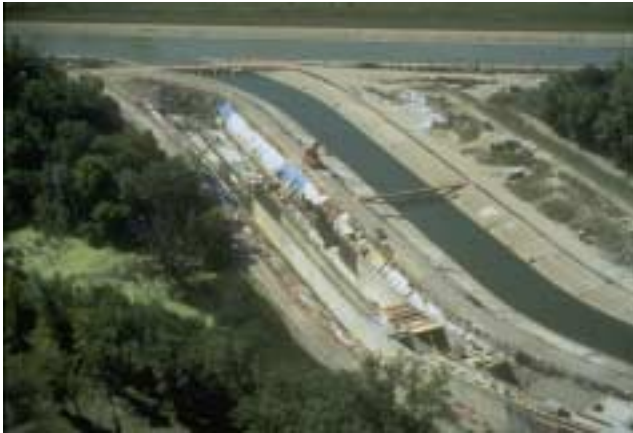
Completed Hubbell-Southfield CSO Facility
