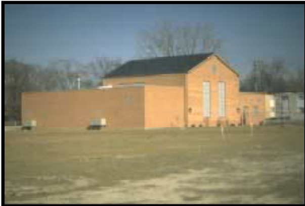
Completed Seven Mile CSO Facility
