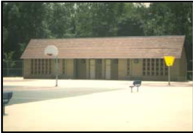
Completed Inkster CSO Facility
