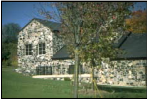
Completed Birmingham CSO Basin
