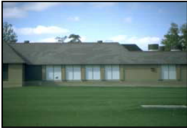
Completed Redford CSO Control Facility
