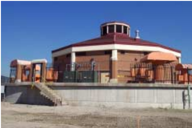
City of River Rouge CSO Control Facility
