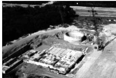
Photo: Retention basin under construction in Dearborn, MI. Courtesy of EPA
