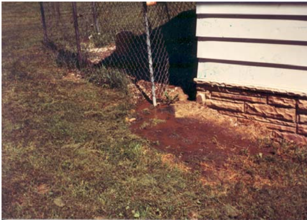
Failing Backyard Septic System
