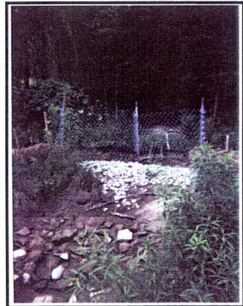
Reinforced gravel check dam upstream of wetland area.
