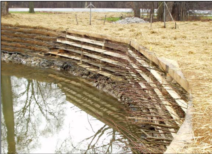
Streambank Stabilization on the Middle Rouge River
