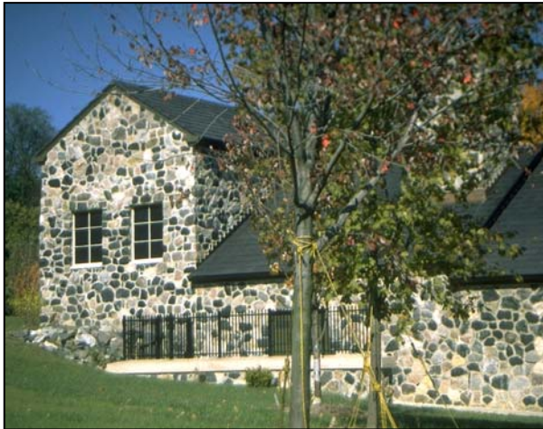
Birmingham Combined Sewer Overflow Basin
