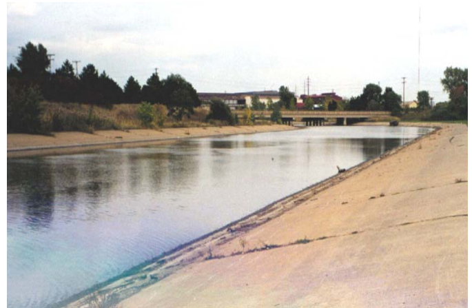
Channelized section of the Rouge River
