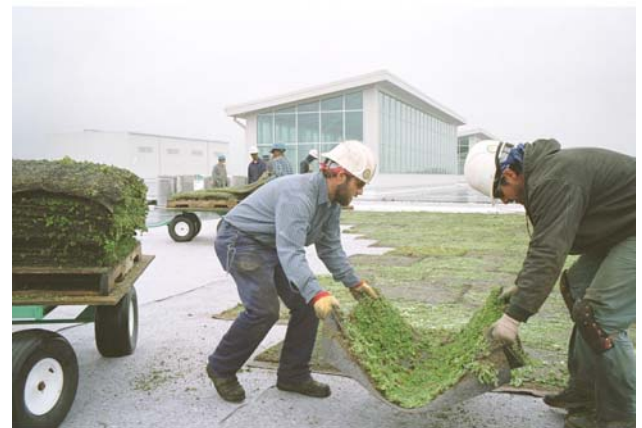
Green Roof Installation at Ford's new Dearborn Truck Plant
