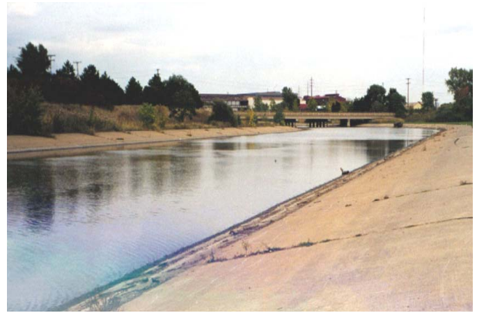
Channelized section of the Rouge River
