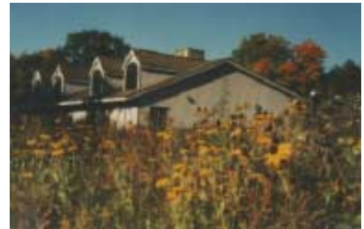
CSO basin at Douglas-Evans Nature Preserve
