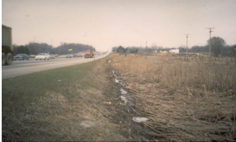
Grassy swale constructed adjacent to interstate highway Upper Rouge River
