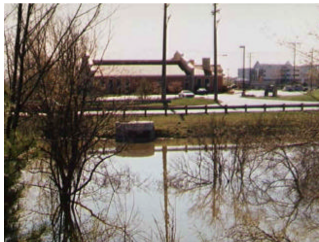
B. Storm water detention area adjacent to commercial development Northville Township, Upper Rouge River
