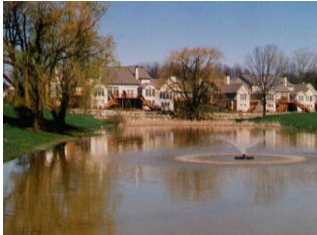
A. Storm water detention pond in residential development Northville Township, Upper Rouge River
