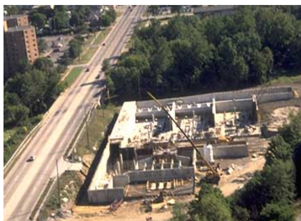
Inkster CSO basin under construction
