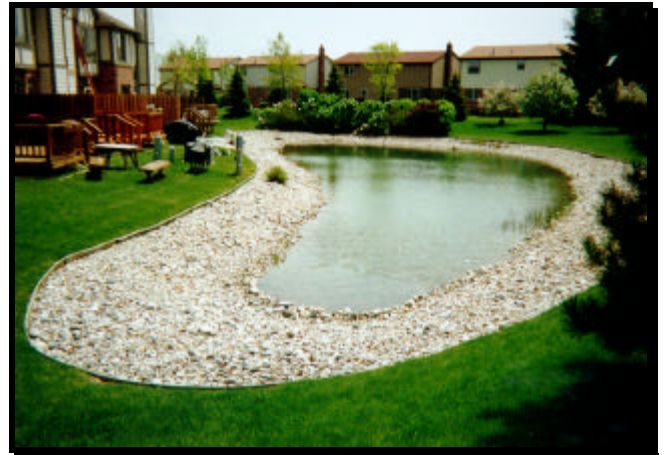
Wet Detention Basin
